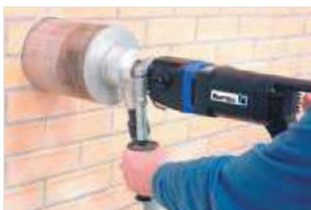
Messa in opera
